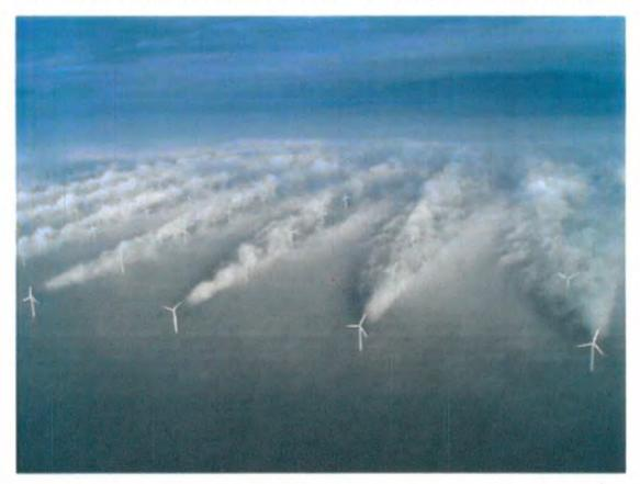
Above shows the impact that "Near" and "Far" wake turbulence will have downwind of wind turbines.
