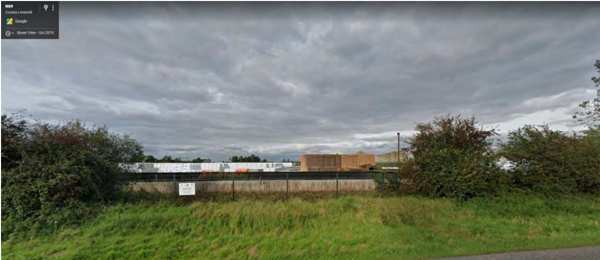
Figure 13 – Street View image from N69 of Goulding site at Askeaton - October, 2019
